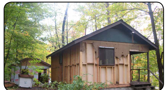
Construction continues on Dutchie's (left) and Sid's cabins.
